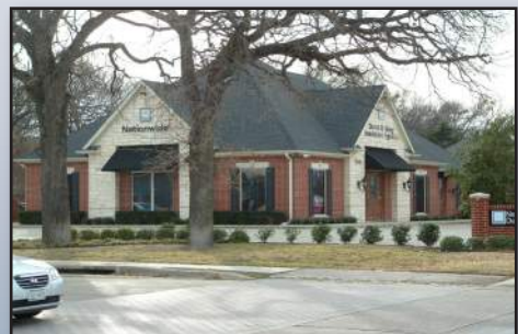
Structures should be architecturally compatible with nearby residential dwellings.
