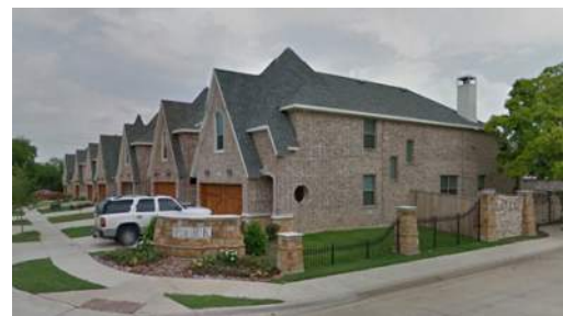
Medium density single family urban residential dwellings (no greater than 10 dwelling units per acre)
