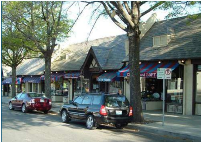
Neighborhoods have convenient access to mixed-use centers with civic spaces and opportunities for social interaction.
