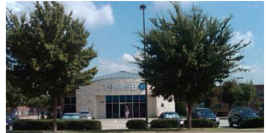
The street level of buildings have a transparent quality for pedestrians and vehicles. Parking is provided both on-street and to the rear of buildings.
