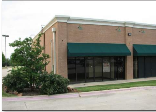
Existing conditions include a number of vacant retail and restaurant spaces.
