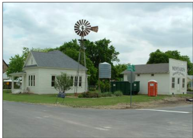
While there are exceptions, most exterior cladding consists of horizontal clapboards. The predominant roof form is the gable, with some buildings including a parapet wall that masks the roof as viewed from the street.
