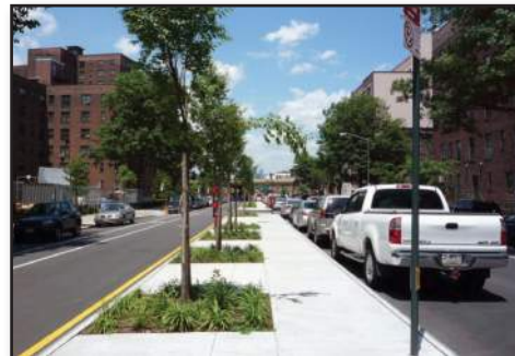
This multi-way boulevard concept in a mixed-use urban environment provides on-street parking and a sidewalk with “green” solutions within the median. Credit: NY Street Design Manual , NY DOT
