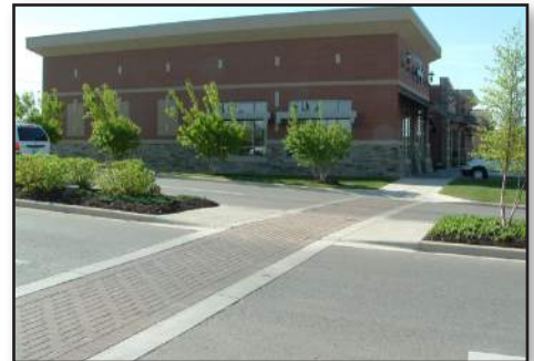
Material changes help define pedestrian crossings through streets and driveways, and also help slow vehicular speeds.
