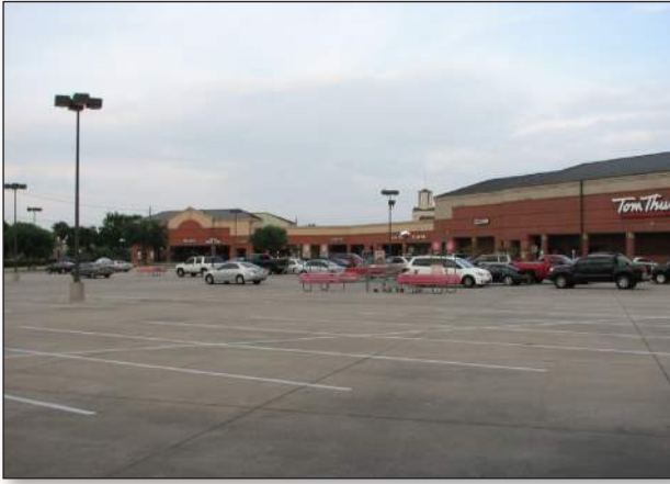
Existing low density retail areas while mostly occupied have large surface parking lots that are underutilized.
