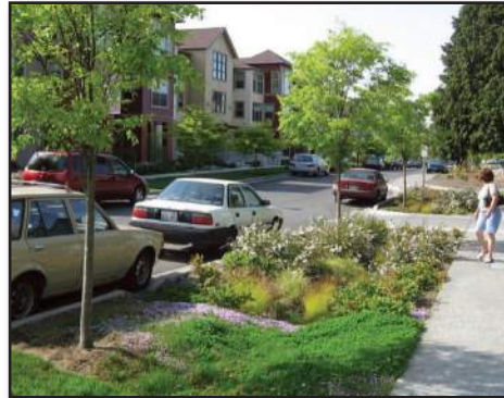
This “green” street in Seattle has a vegetated swale between the street edge and the sidewalk, providing natural drainage and filtering of storm water in a residential area. Credit: NY Street Design Manual, Abby Hall
