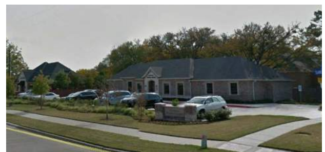
Buildings are compatible with surrounding neighborhoods.
