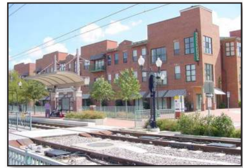
A transit station is supported by higher density development within walking distance.
