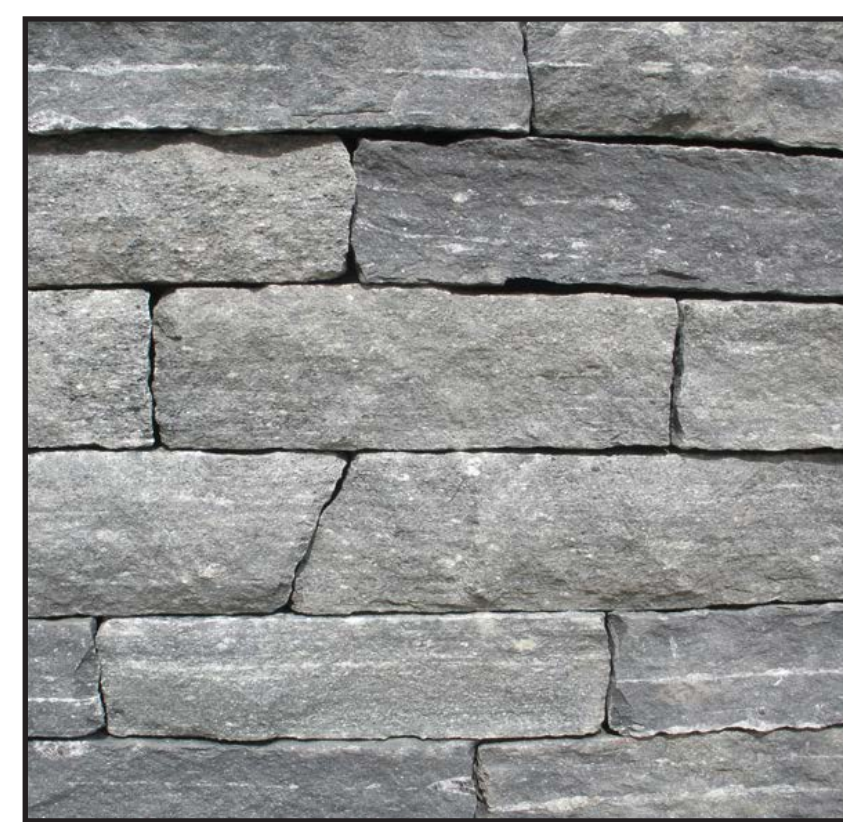
2 Primary Building Stone • Greenwich Gray Limestone
