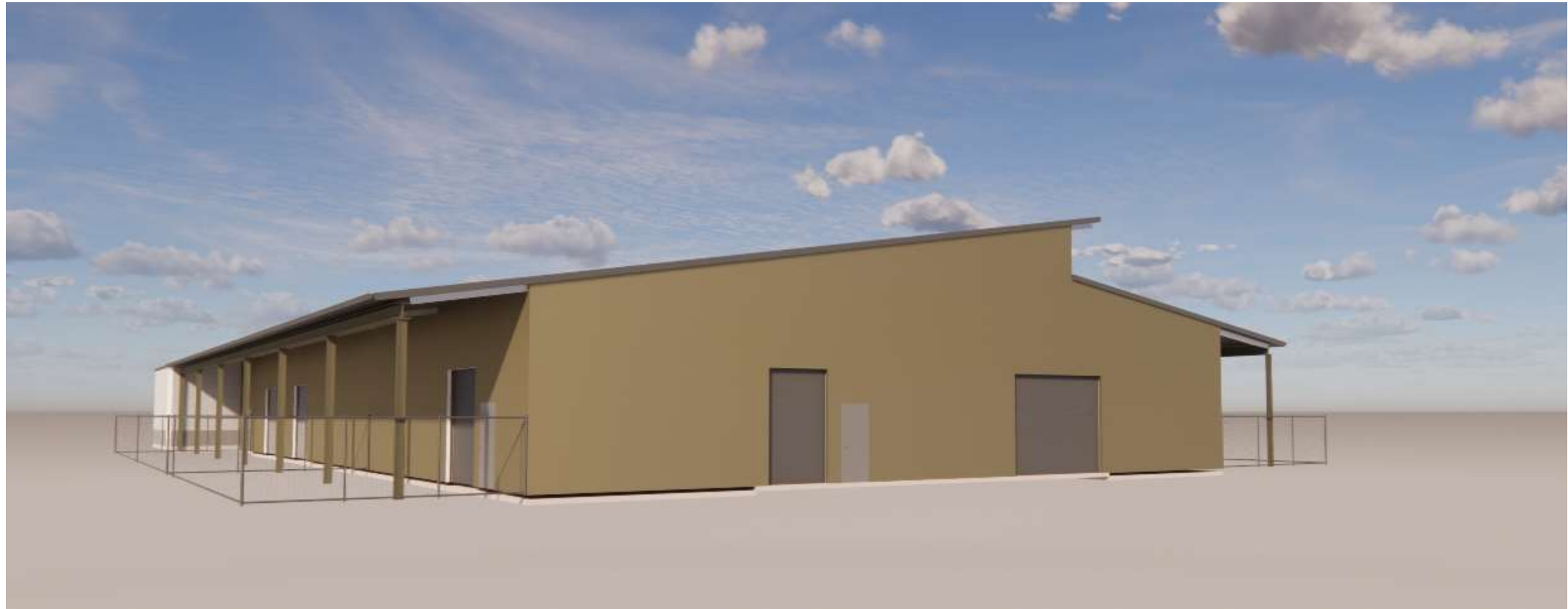
VIEW FROM NORTH EAST CORNER LOOKING SOUTH
