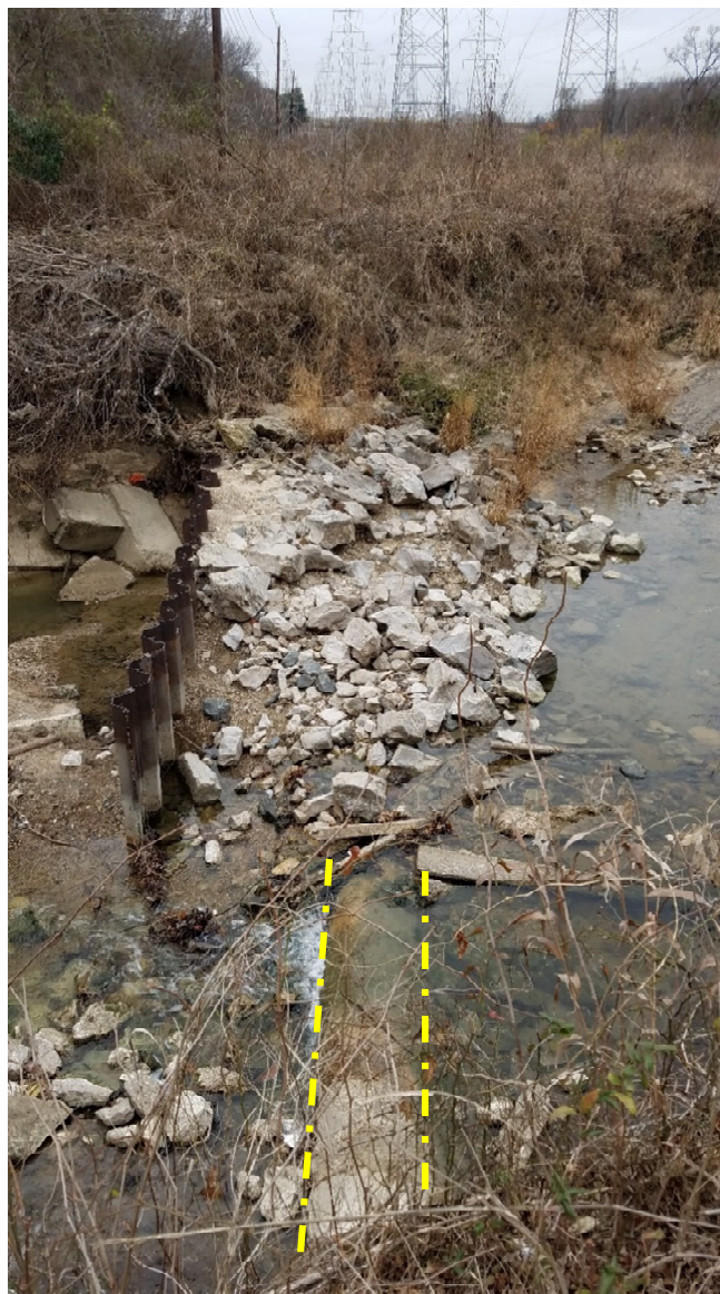
Figure 7.9: Exposed Pipe at Grapevine Creek Crossing Facing West
