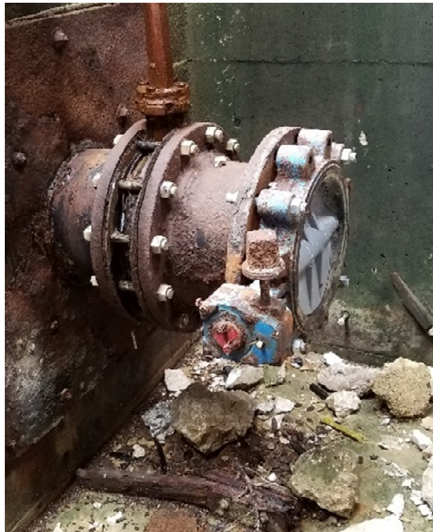
Figure 7.11: 12-Inch Butterfly Valves Near Bottom of Wall
