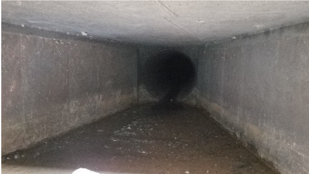
Figure 7.10: Trapezoidal Flume-Like Structure at Outfall Structure
