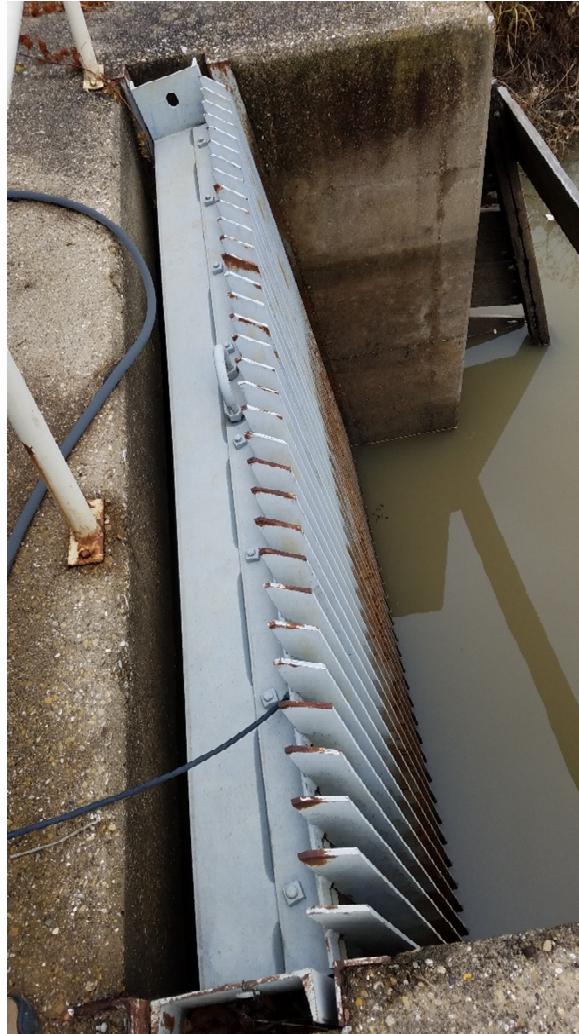
Figure 7.2: No. 3 Pump Bar Screen
