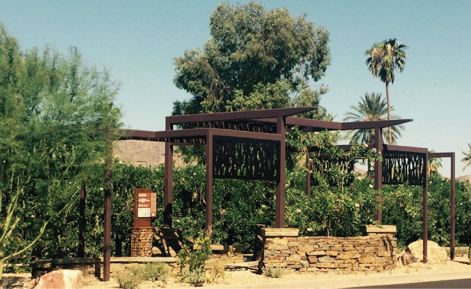
Completed shade structure and signage (primary node)
