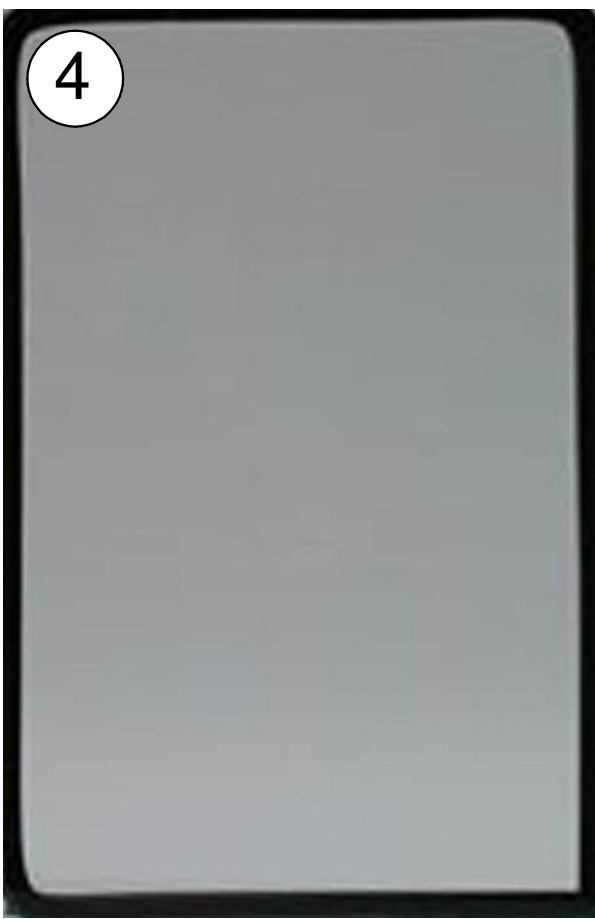
4 GLAZING - 1" INSULATED LOW-E TINTED GLASS
