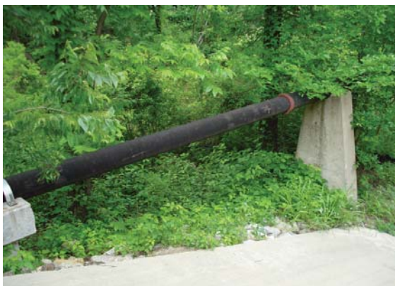
Exhibit C.3 Exposed Utility at Bridge
